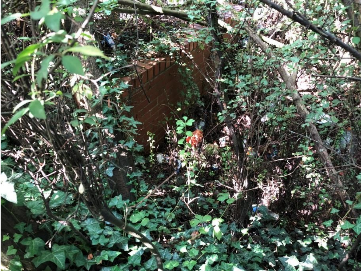
Culvert entry from Grangewood Park
