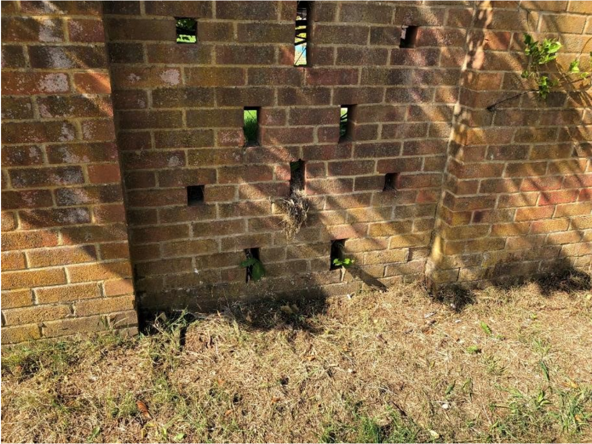
Wall to rear gardens of Swallow Close
