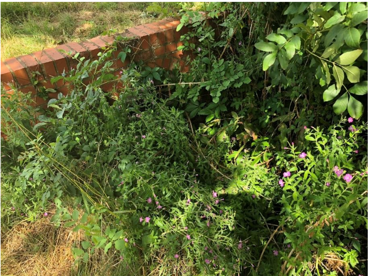
Culvert entry from Penvale Park watercourse
