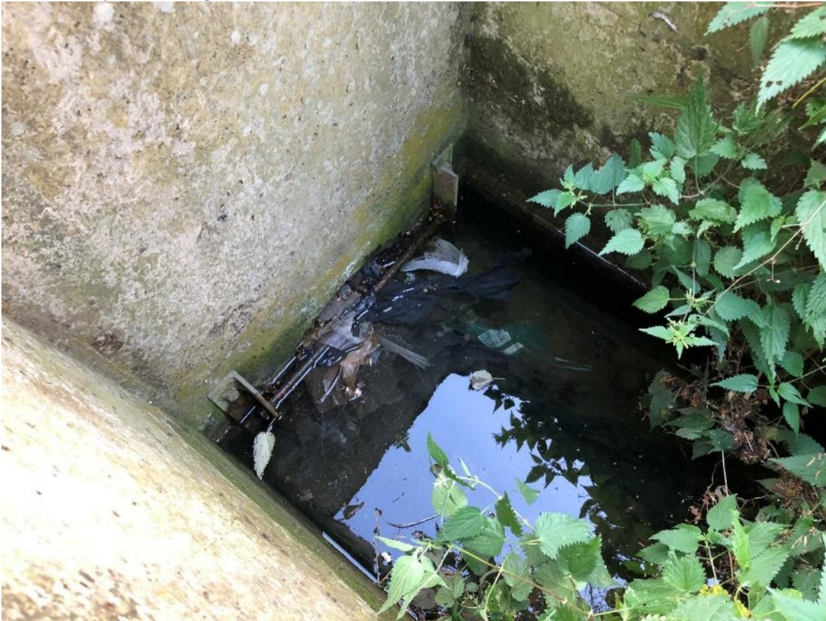
Culvert exit (south of Swallow Close)
