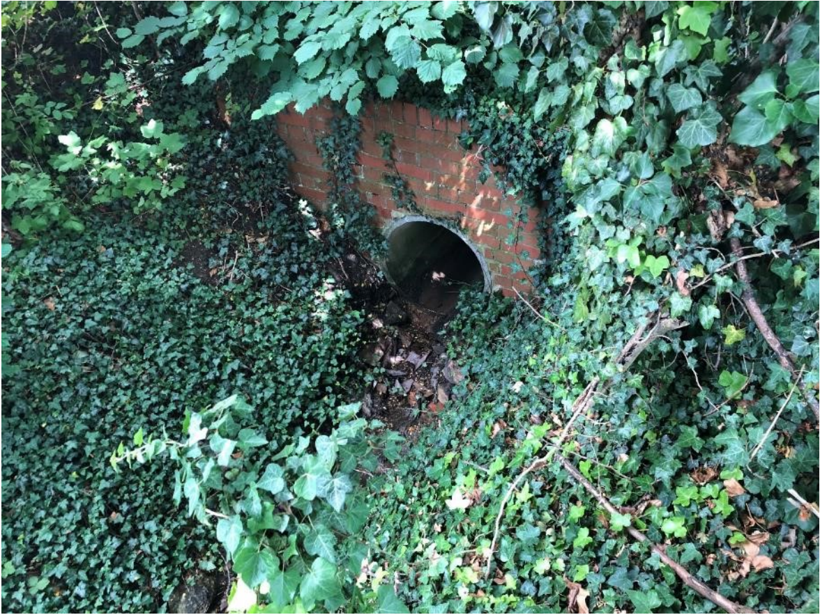
Culvert exit (Hilldrop Road)
