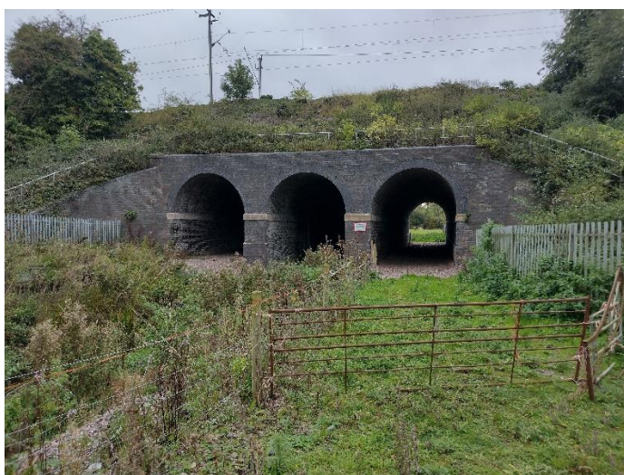
Tunnel entrances – Western expansion site to Towcester Road
